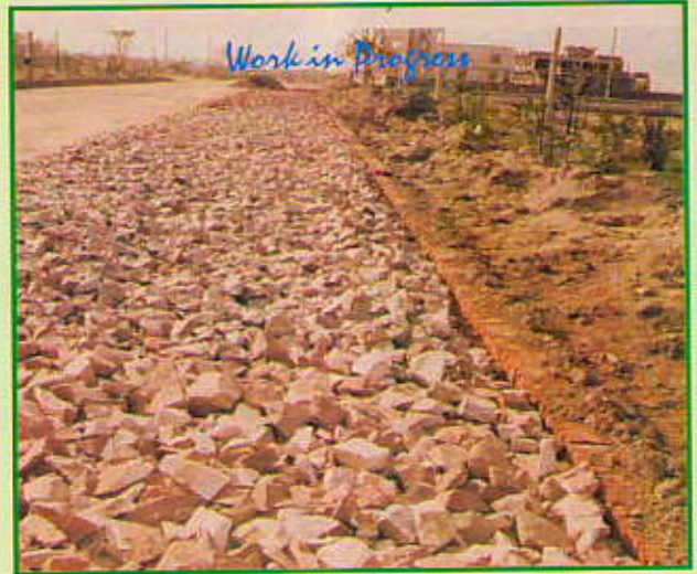
WIDENING 45 MTR. ROAD PHASE-II, NOIDA
